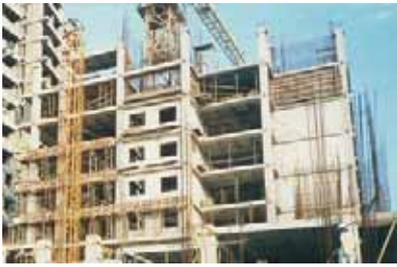
**Stiffening walls** (M 40) are reinforced concrete panels (minimal depth – 15 cm), which stiffen the frame. They are positioned, by the rule, in the axis of two adjacent columns, having a function to form, together with columns, a structural element from foundations to the roof, ready to receive required intensity horizontal forces (in practice, those elements are often set in concrete in situ, especially at larger spans for the reasons of huge dimension, weight and slow frame erection).
