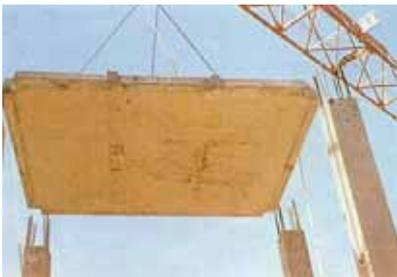
**Cantilever floor slabs** (M 40), which replace edge beams in architectural solutions where balconies, loggias or other housing space out of column span are required and which are connected only to two columns (as a cantilever) and their height and length correspond to floor slabs near which they are erected, while their maximal width is limited on 1/3 of the longitudinal span. They are waffled and can be with or without concrete ceiling.
