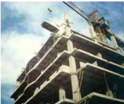
**Edge girders** (M 40) have a boundary position in order to form frame beams and facade construction. Their lengths and depth are the same as at corresponding floor slabs with which they form a frame beam and their width is chosen according to architectural requirements for the adequate type of facade walls.
