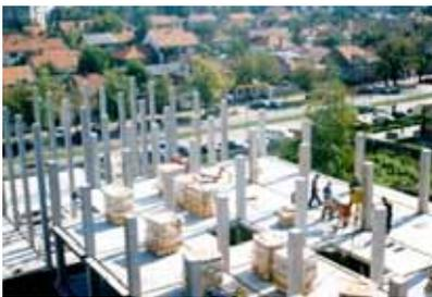
**Floor slabs** (M 40) cover space between columns and can be manufactured with or without concrete ceiling, as one-piece (spans until 3.6 x 4.8 m) or multi-pieces aiming to adapt dimension for transportation and erection (ceilings made for the span 9.0 x 9.0 m are constructed from nine standard elements); the marginal girder and waffle web height is 20-40 cm (depending on column span between which space is covered), floor slab depth between coffer webs is 4-6 cm, and the ceiling one is 3cm.
